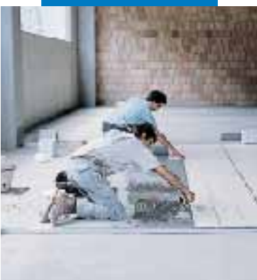
Laying porcelain tiles in a factory
